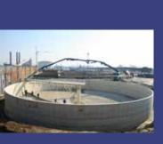
"The floor of settlement tanks is cast at a gradient as specified by the customer"
