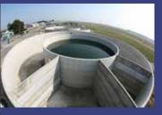
"Aeration tanks are usually constructed at a height of 7 m to 10 m to ensure the most efficient absorption of oxygen"
